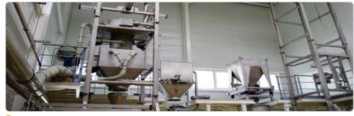
🜔 Unloading solution: FIBC, bag, container (semi-automatic, containment, ergonomic, ATEX dust collector, loss-in-weight stations, big bag massing paddles)
