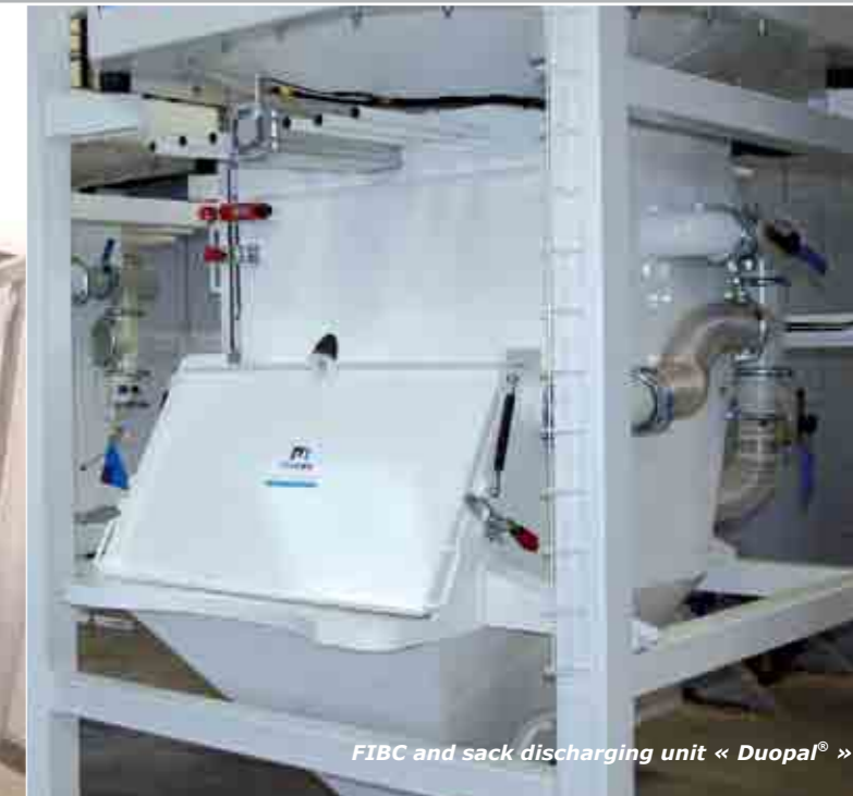
Raw materials deconditioning area
